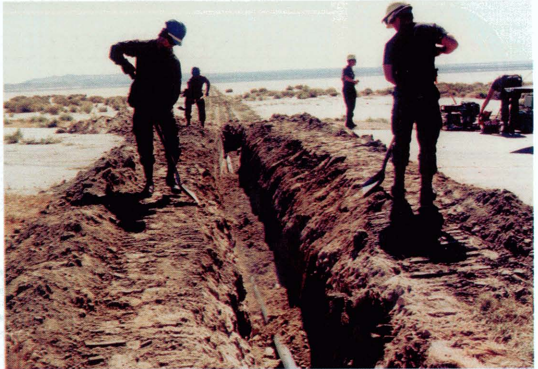
Workers trench across Rogers Dry Lake to install fiber-optic cables.
